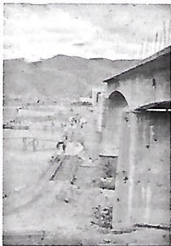
Portion of abutment of original road/rail bridge spanning the Imjin River?
