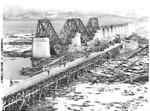
Destroyed Imjin River Bridge 1950 and replacement 'full service' bridge being constructed by U.S. Army Engineers, o/a late Oct 50.
